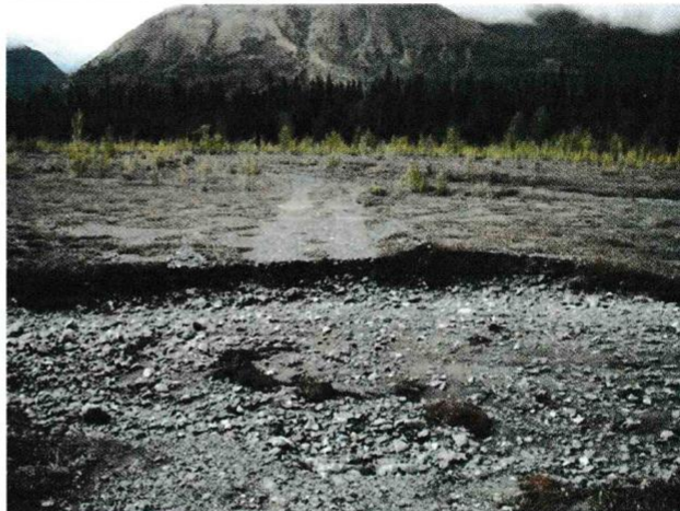
Plate 1: Washout on access trail
